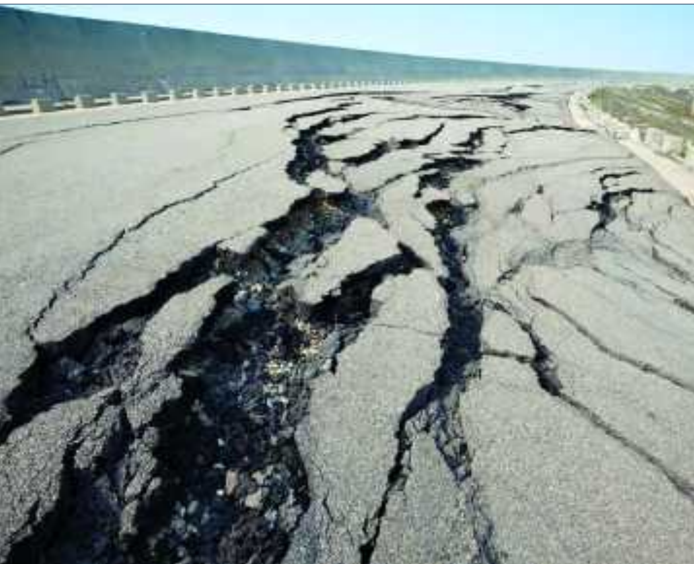
Cracks in the roads – the consequences of the earthquake
