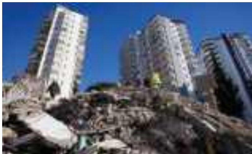
Fig.4. Destroyed building in Kahramanmaraş
